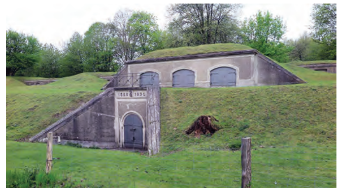
Gun Battery with associated underground magazines at Vestvolden. The guns themselves were kept nearby under cover apart from exercises and hostilities
